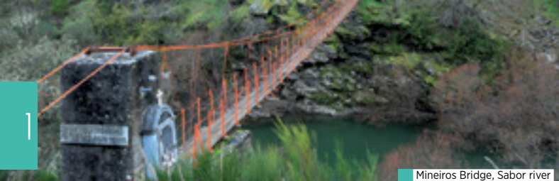
Mineiros Bridge, Sabor river
